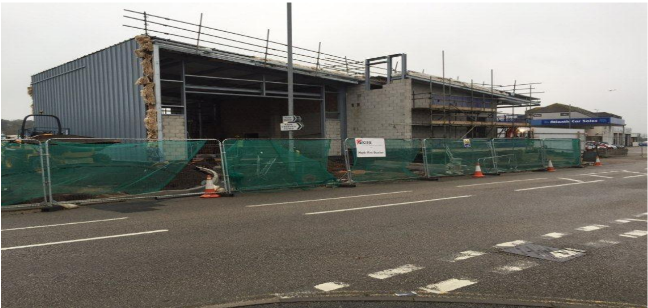
Hayle, Tri-partite Emergency Services Base in construction, 2015
