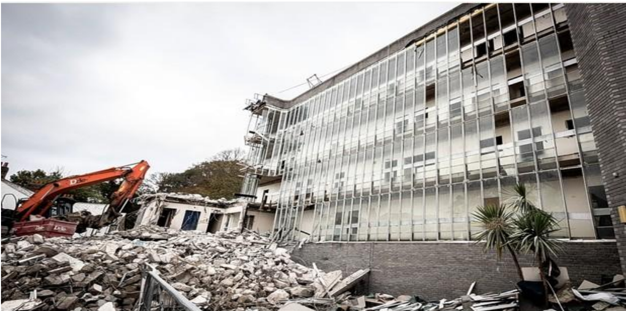
Truro Police Station, demolition of Tregolls Road 2015
